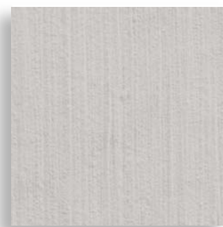
Brush Finished TILT-UP CONCRETE WALL
